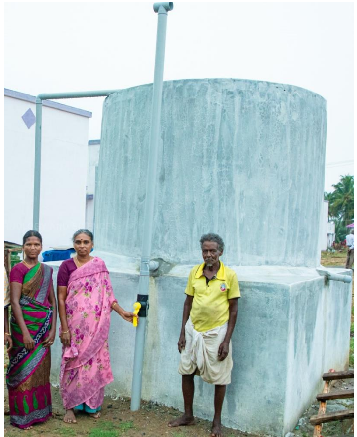
Ferrocement Tank for Drinking Water – Rural Water Supply
