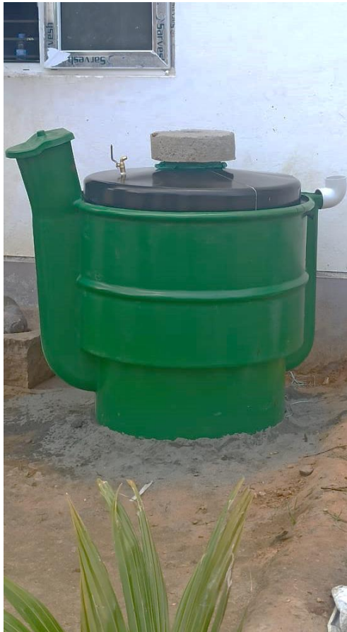
Household Biogas plant
