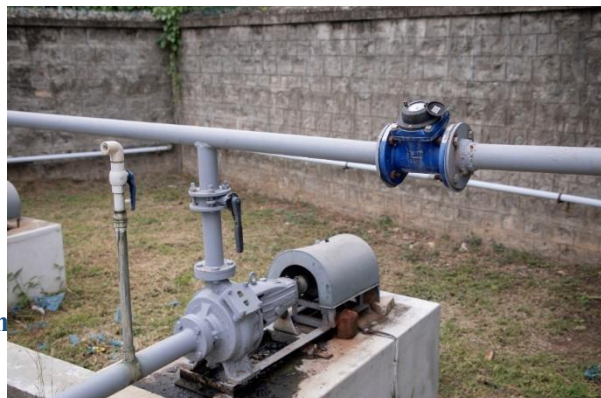
Flow Meters at the Filter Unit of Treatment Plant to measure the Treated Water
