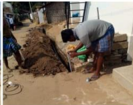
Installation of pipe line
