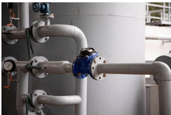
Flow Meters at the Filter Unit of Treatment Plant to measure the Treated Water
